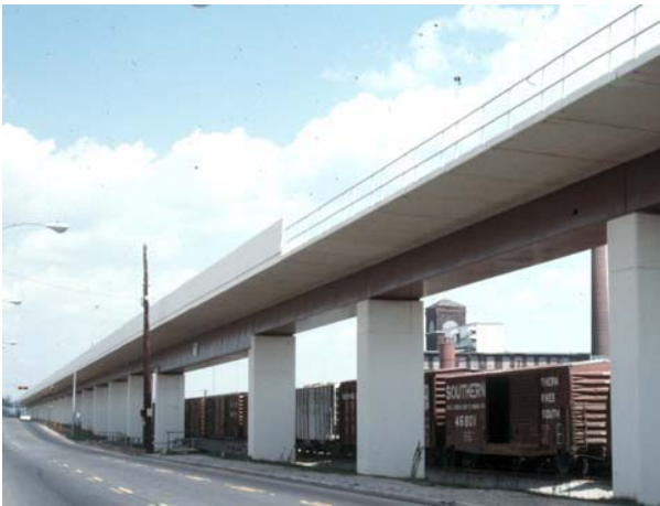
Figure 5 MARTA double track concrete deck with damped steel girder and sound barrier wall
