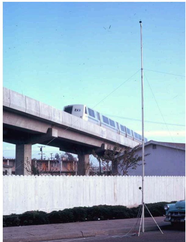
Figure 4 BART concrete viaduct with sound barrier wall
