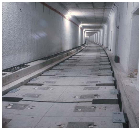
Figure 8 Photo of TTC double-tie system in subway - before installation of the rail fasteners and rail.
