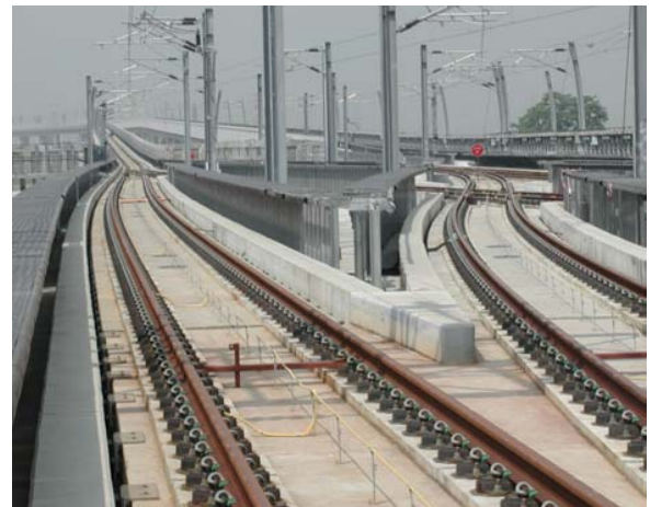
Figure 10 Photo of KCRC viaduct completed
